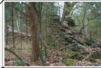
Fallen chimney, mid-late 1800's
