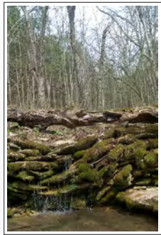
Old dam, probably built by Luttrell family in 1800's
