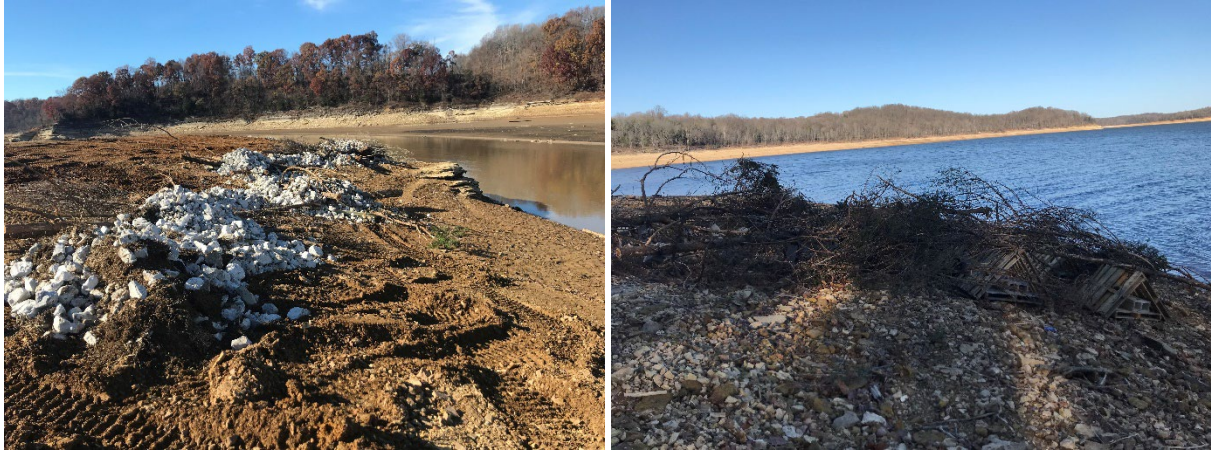
Figure 1 (left photo). Spider-hump construction at Beaver Creek. Figure 2 (right photo). Brush pile material made of large cedar trees and wooden pallet structures at Peninsula Marina area, Phase 4 and 5.
