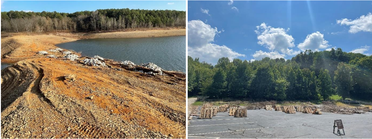
Figure 1 (left photo). Spider-hump construction near Peninsula. Figure 2 (right photo). Brush pile material and wooden pallet structures staged for deployment at Peninsula Marina area, Phase 6.
