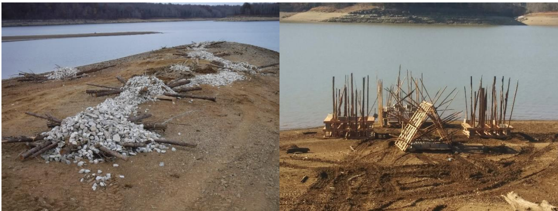
Figure 1. (left photo). Spider-hump construction during drawdown. Figure 2 (right photo). MEGA stake-bed structures placed during drawdown.
