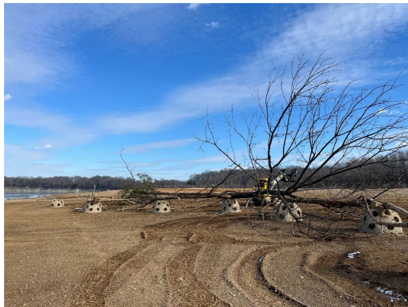
Figure 12. Photo of reefball site at Barren River Lake. Reefballs were dropped during high water at summer pool, then trees were tied between the reefballs during low water at winter pool. Another example of a technical guidance project. This project was done with three days of fieldwork.
