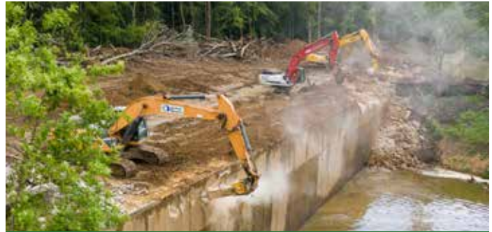
Removal of Green River Lock and Dam #5. Photo: Mike Wilkinson, The Nature Conservancy
