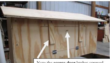
Note the **access door** latches screwed through the **front** into the **access door doorstop** 2"x2". Swing latches out of the way to open **access door**. Note the partially driven screw at the top of the **access door**. Assists with opening and closing.
