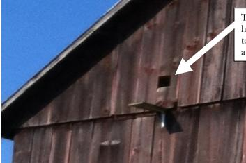
The exterior entrance is a 5-1/2" square hole cut into barn siding providing access to the box. Note the **perch** below attached with a shelf bracket.
