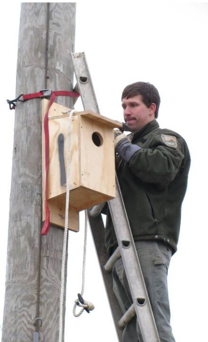
KDFWR staff used a ladder to place this nest box on a retired power pole on a WMA. Galvanized screws hold it securely to the pole. Photo by: KDFWR
